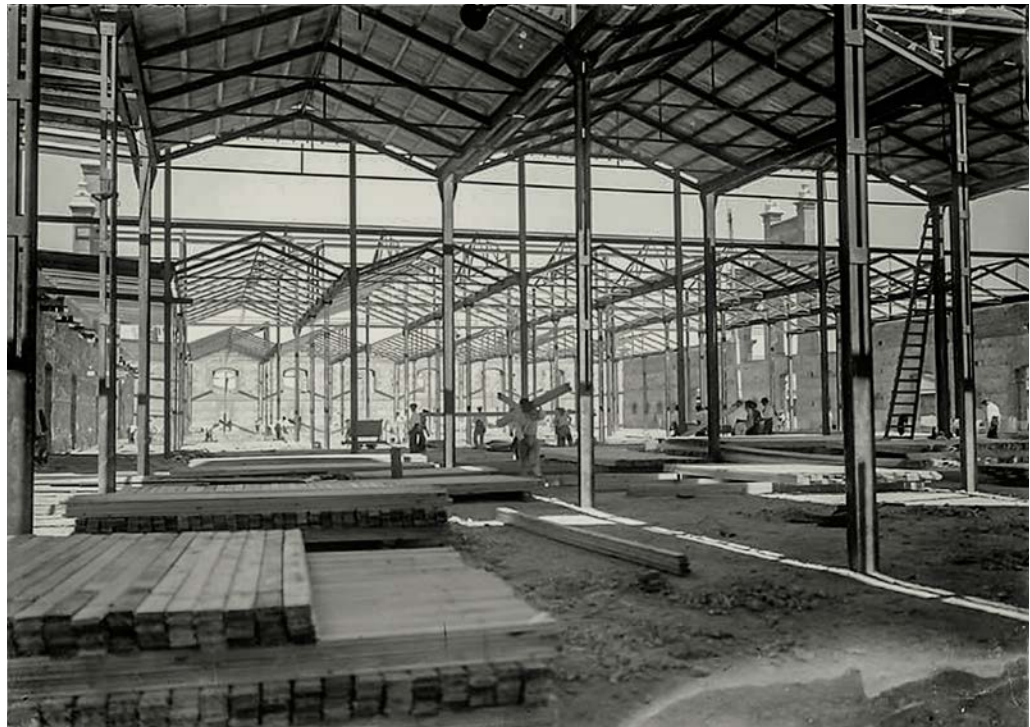
Photo 3. Works in the warehouse for the exhibition, selling and housing of pigs in the municipal slaughterhouse, 1916. Publisher: Servicio Fotográfico Municipal. The photograph shows the construction technique and materials used. CC. Biblioteca Digital Memoria de Madrid.
