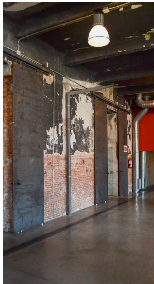
Photo 5. Intervention of the interior of warehouse 17c of Matadero (Anteroom to Intermediæ and the Central de Diseño). September 2018. Author's photo.
